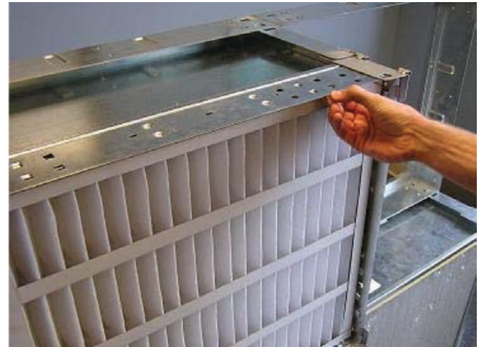
Figure 31: Installation of Prefilter into Frame
