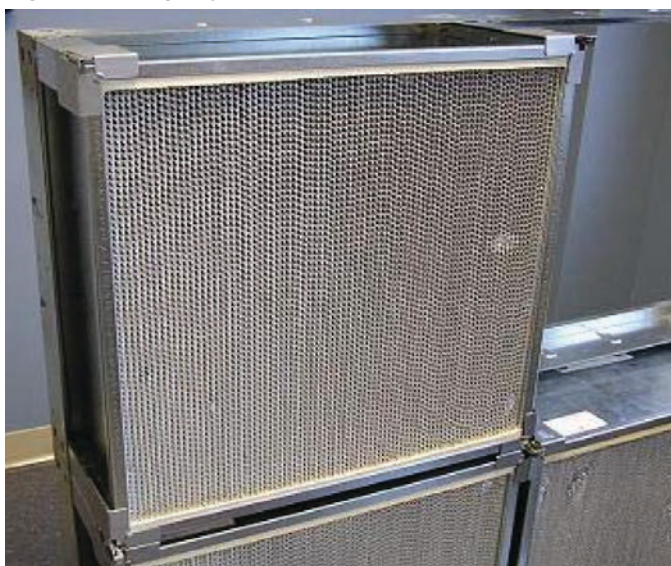
Figure 25: Properly Installed Filter Inside of the Frame
